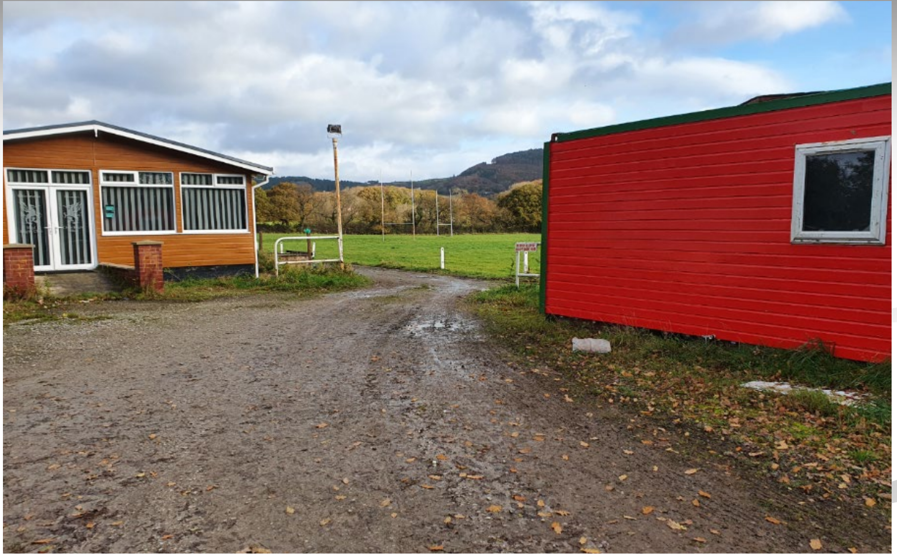
View of existing buildings
