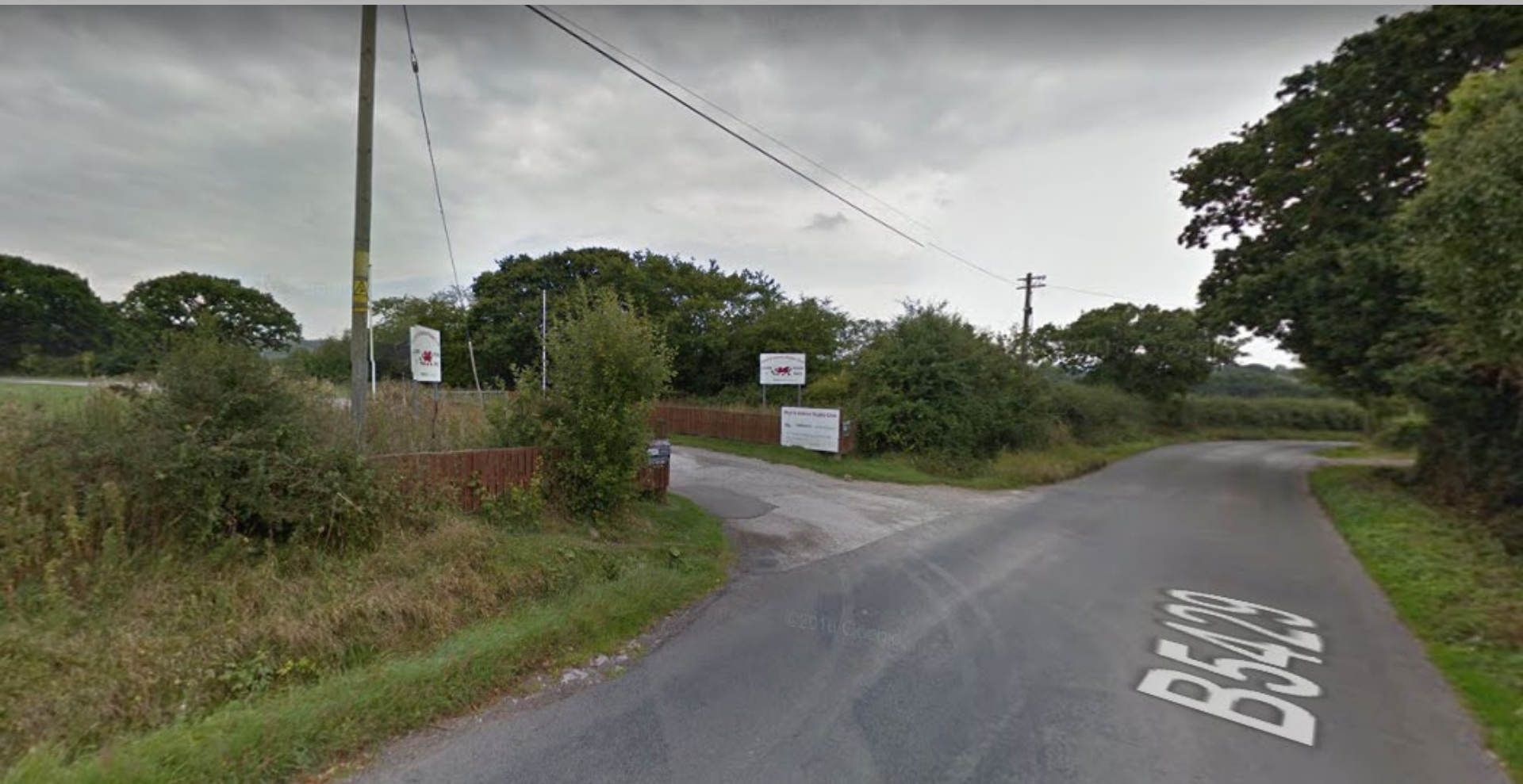
View from along highway (google streetmap)
