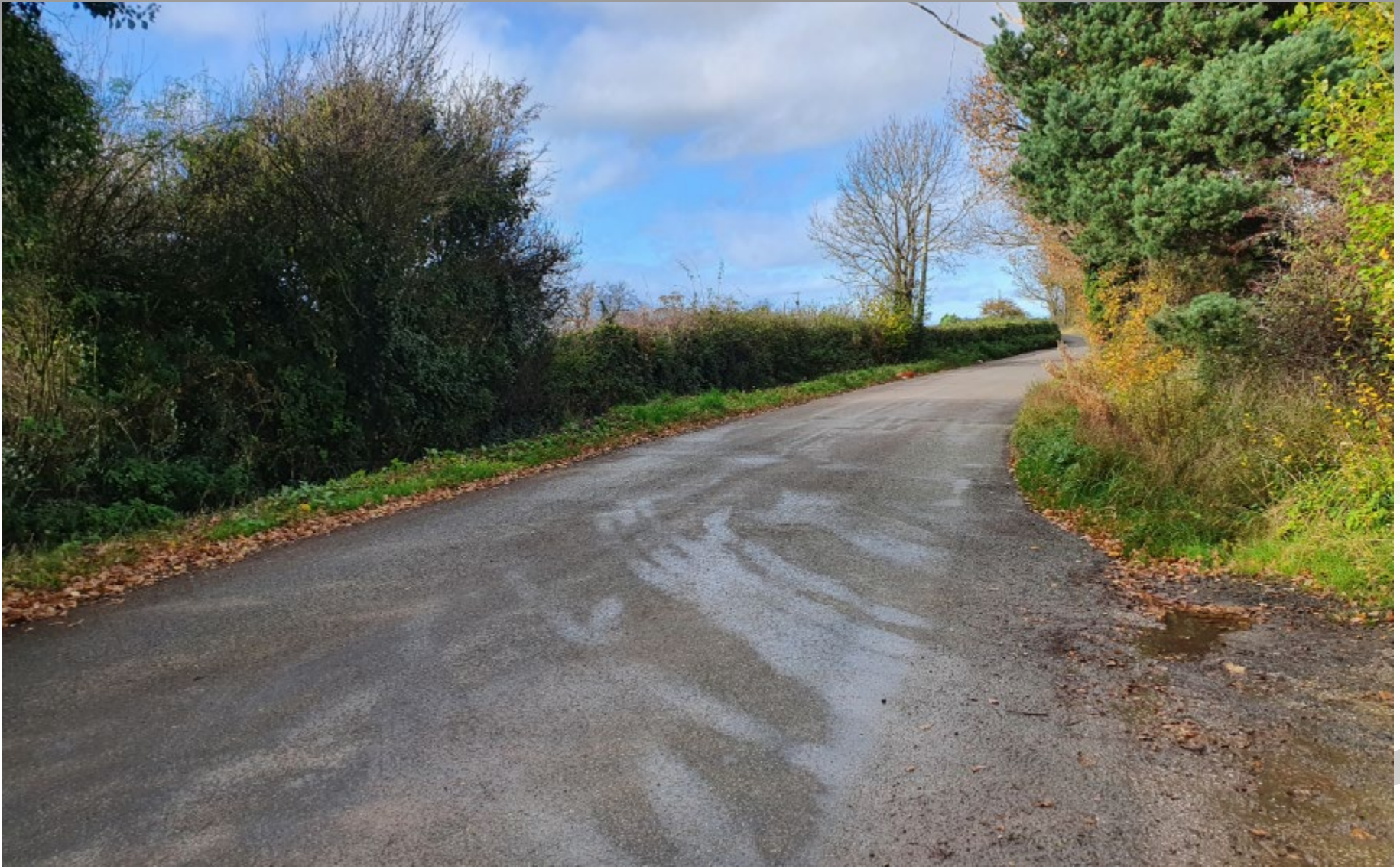
View along highway to the north
