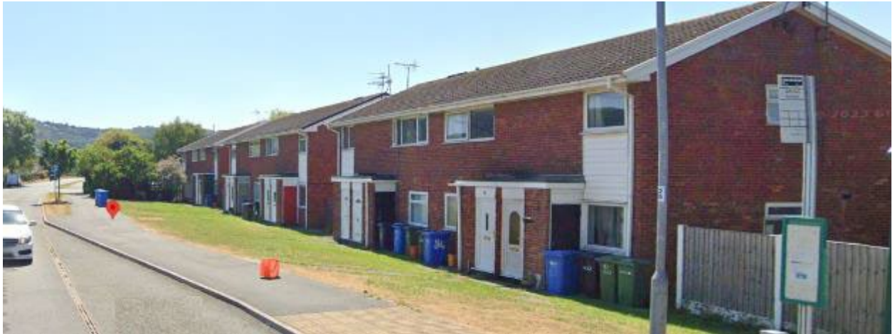
Photo 7: Photo showing the drop in gradient in front of the flooded ground floor flats at Ffordd Penwhylfa
