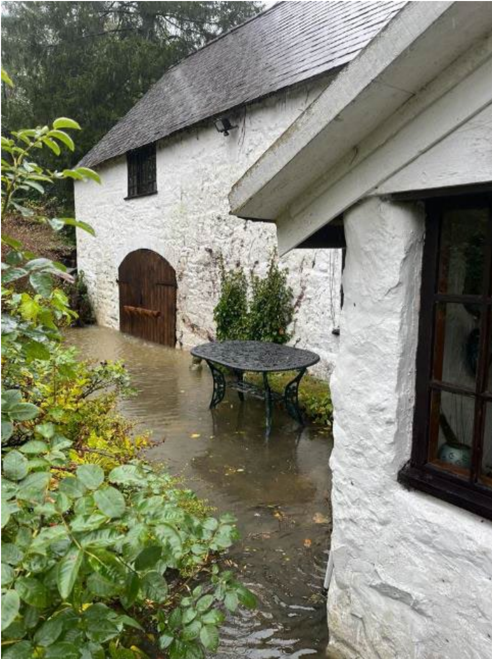
Photo 11 showing flood waters at the front door of Plas Isaf
