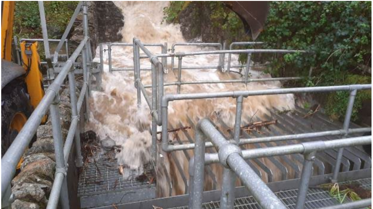
Photo 12: Flood Alleviation Culvert below Pen y Pigyn at Corwen during Storm Babet
