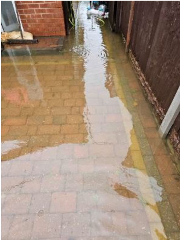
Photo 5 – Flooding at No 1 Winchester Drive
