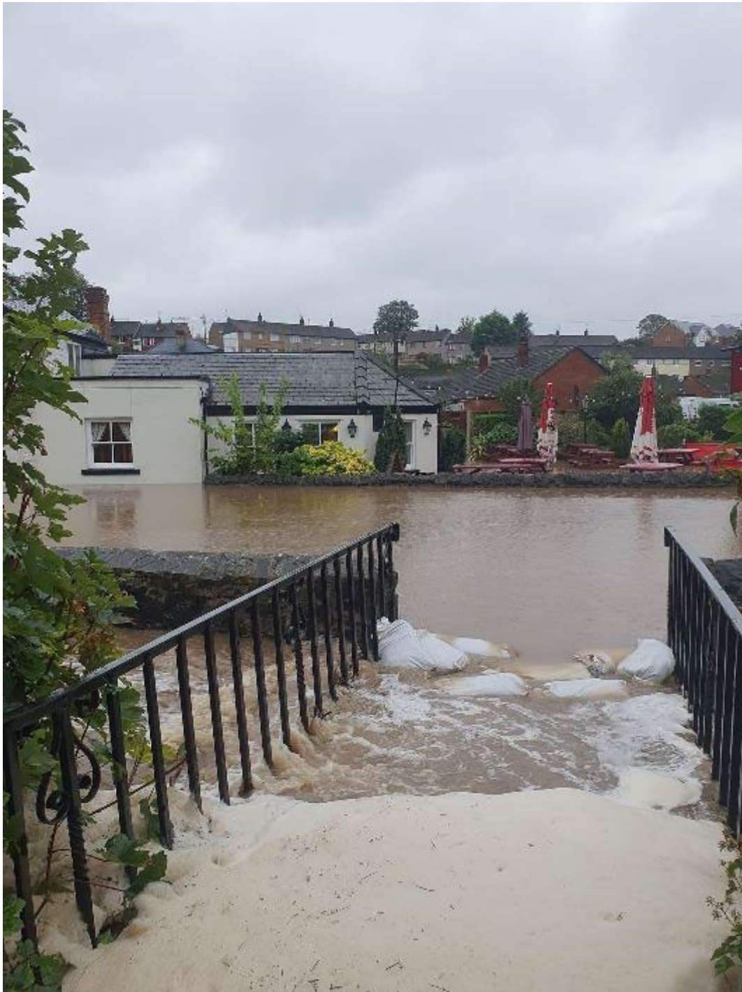
Photo 8: Flooding from the Afon Ffyddion onto Waterfall Road
