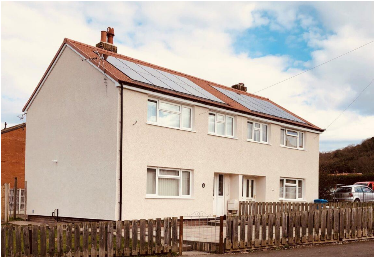
Figure 2.0.1: Rooftop solar PV in Meliden, Denbighshire
