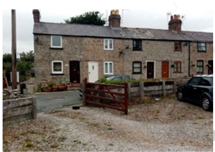
Site Photos – Rear and Front
