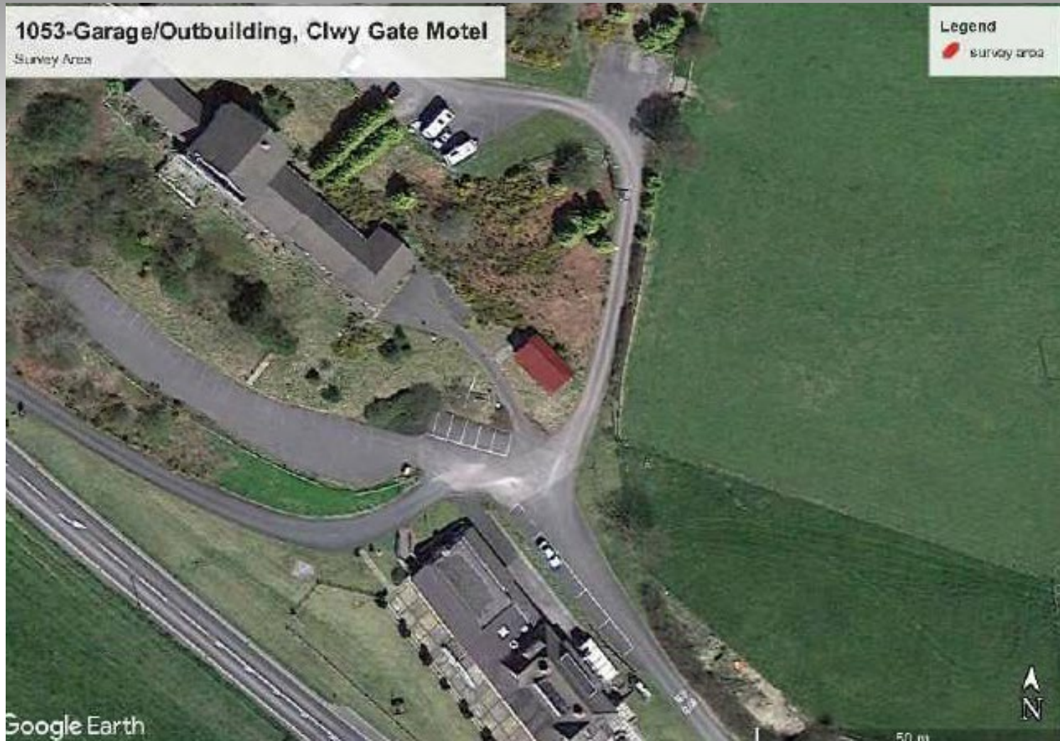
Aerial view of site- former generator building highlighted red
