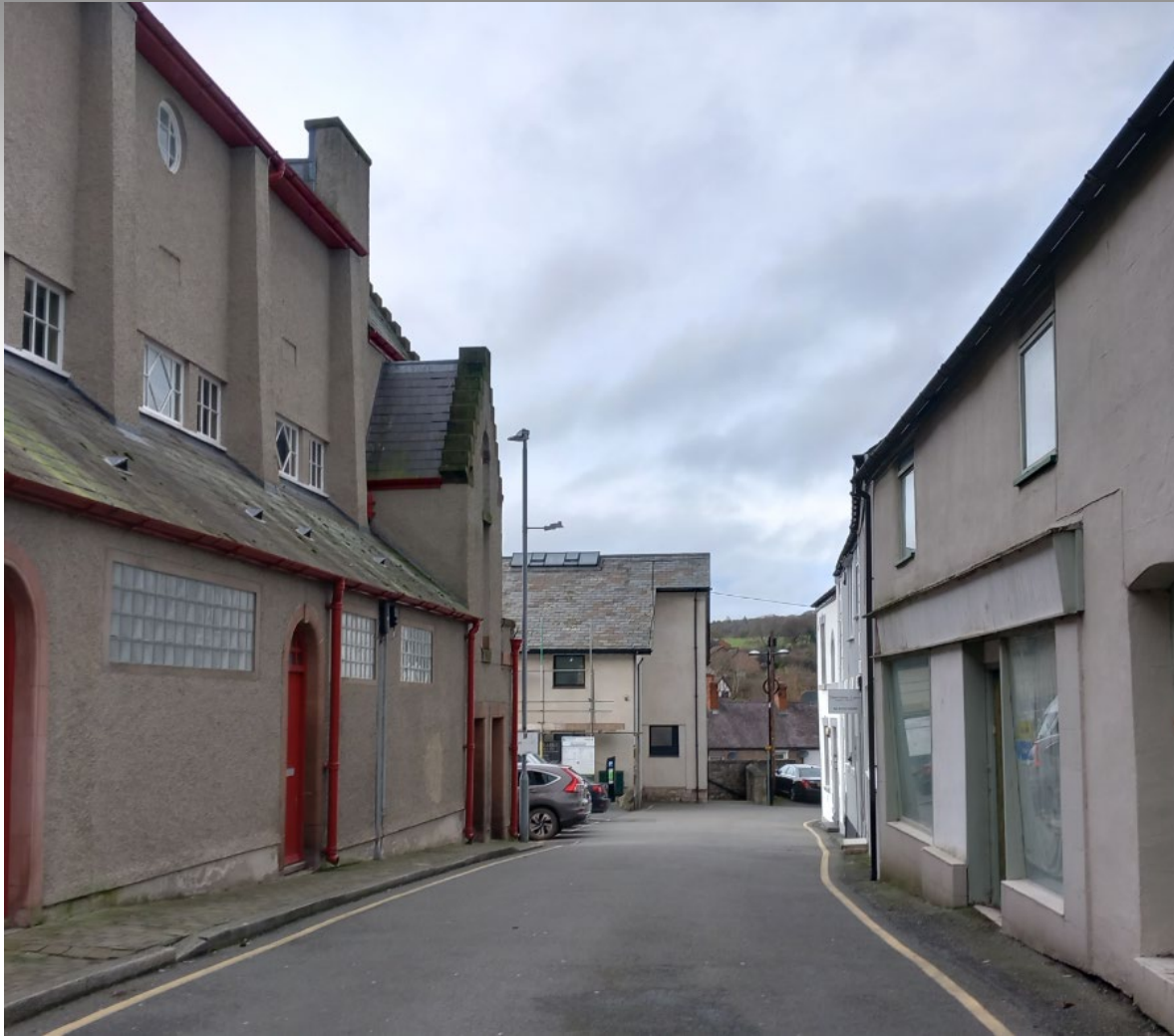
View from corner of Town Hall down Crown Lane
