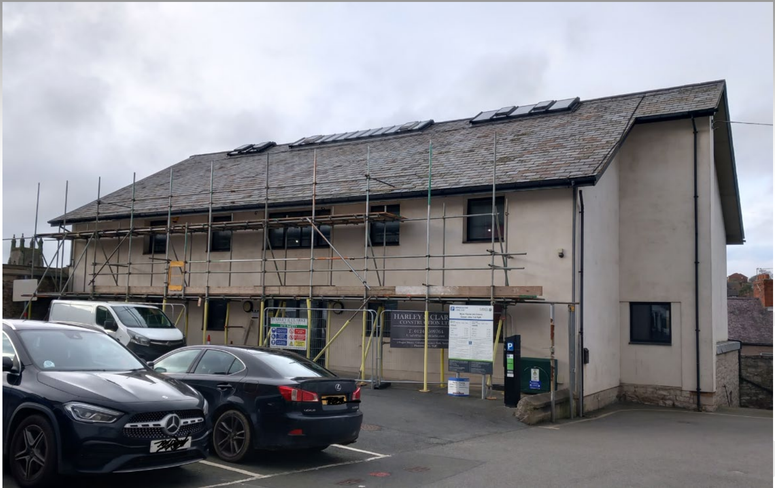
View from rear car park behind Town Hall
