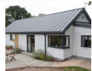
Silicone render with standing seam roof
