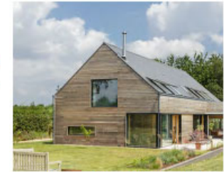
Horizontally laid timber cladding
