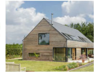
Horizontally laid timber cladding
