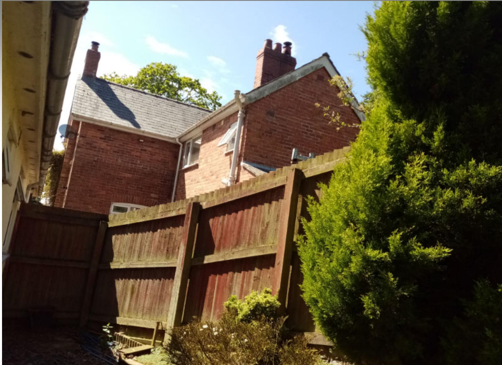
View from side elevation of neighbour's property
