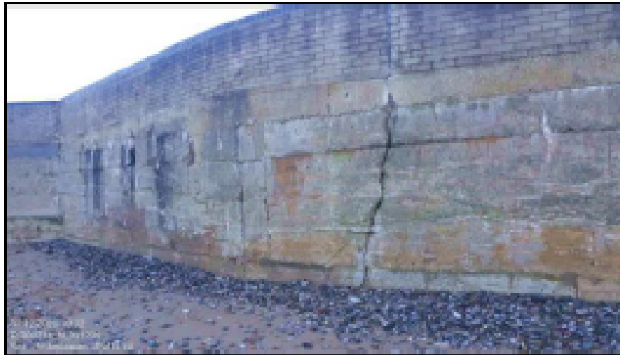
Figure 1.2: Deteriorating defence condition along the Rhyl frontage
