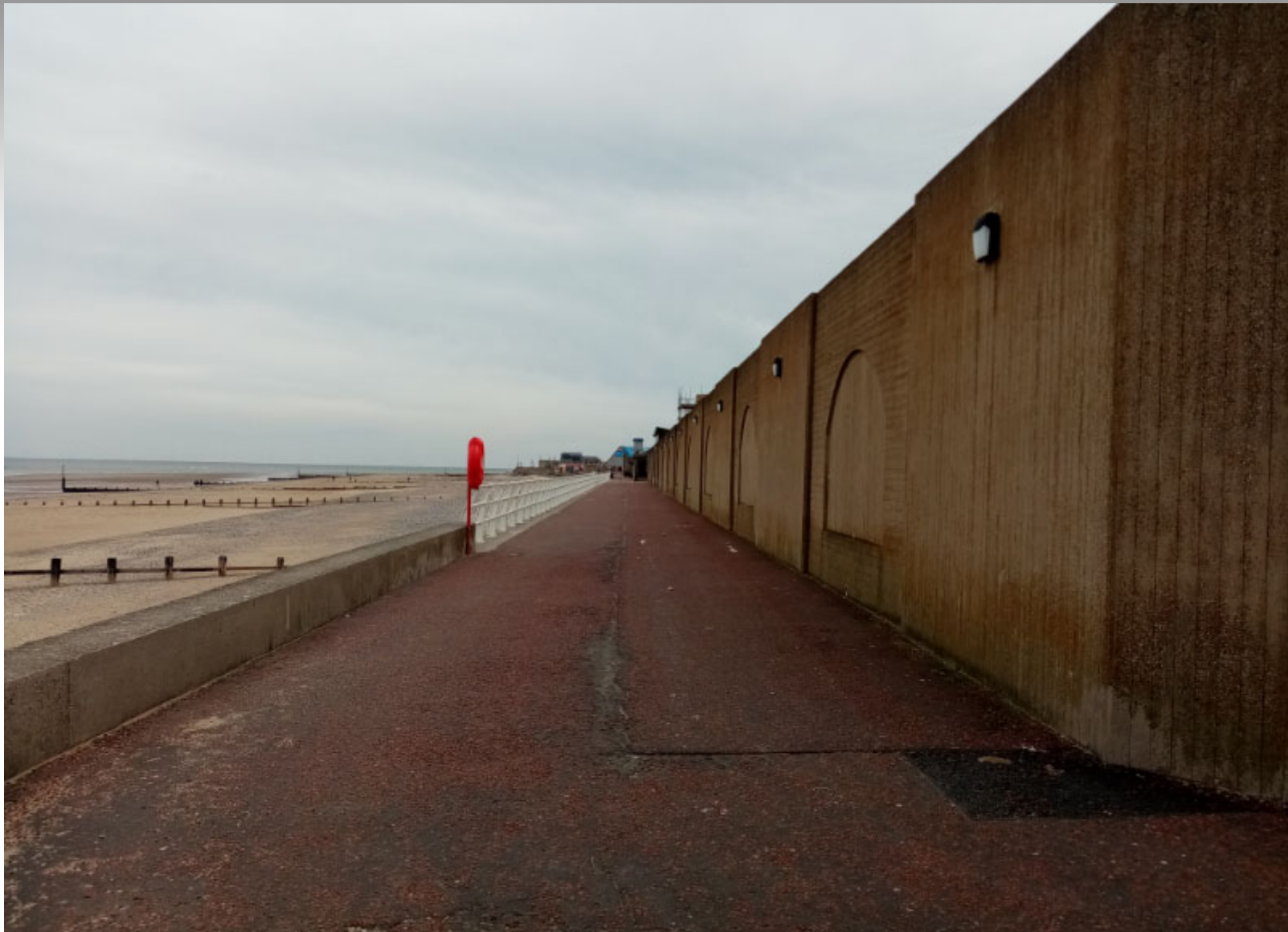
Existing promenade and defences
