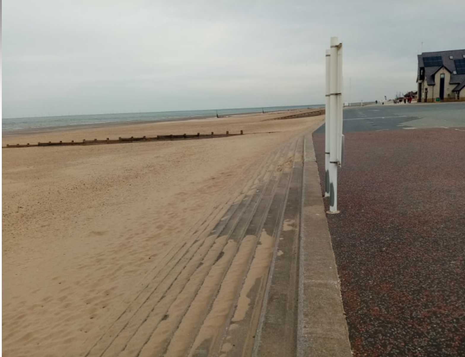
Existing promenade and defences
