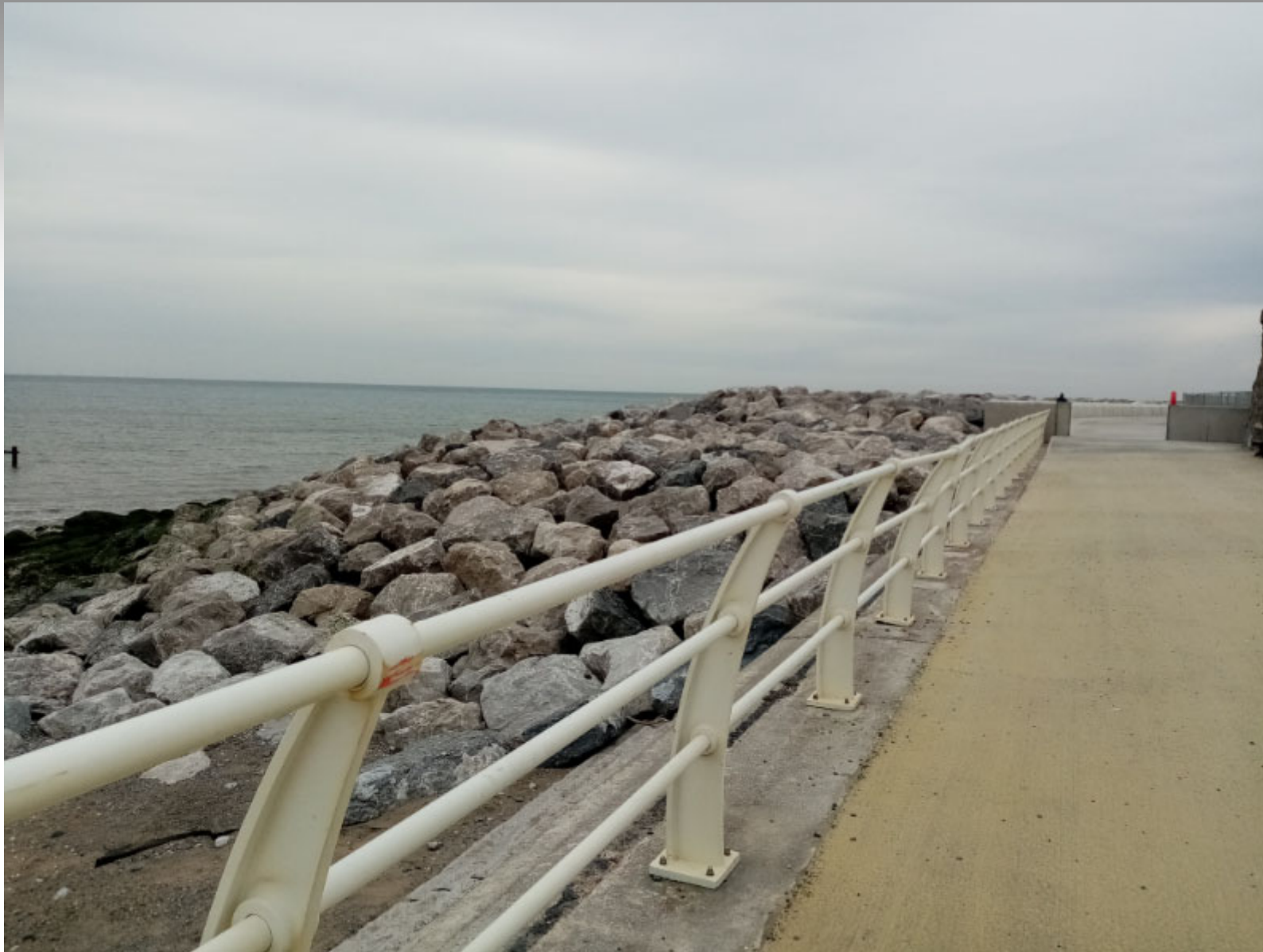
New East Rhyl coastal defences (rock revetment) at Splash Point
