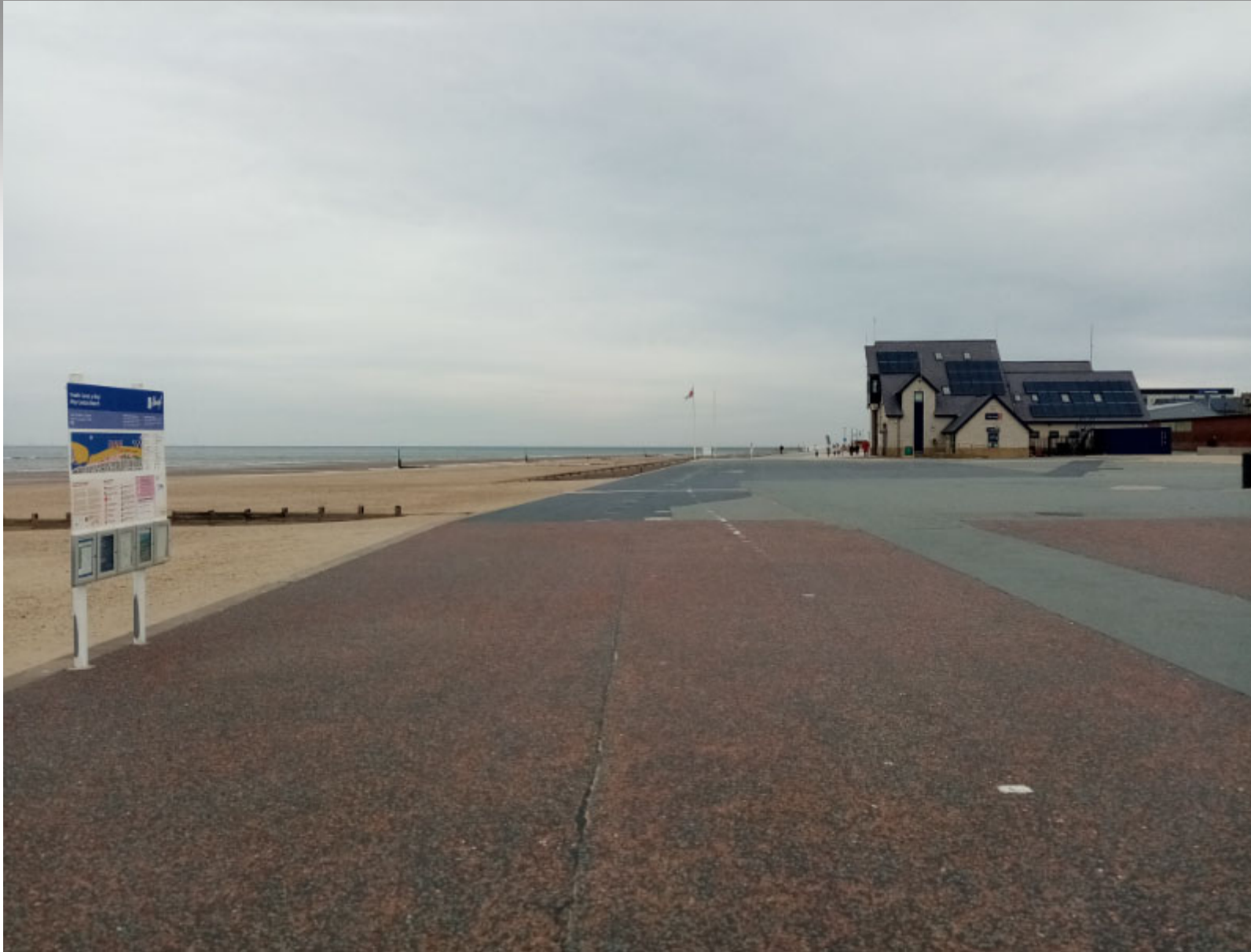
Existing promenade and defences
