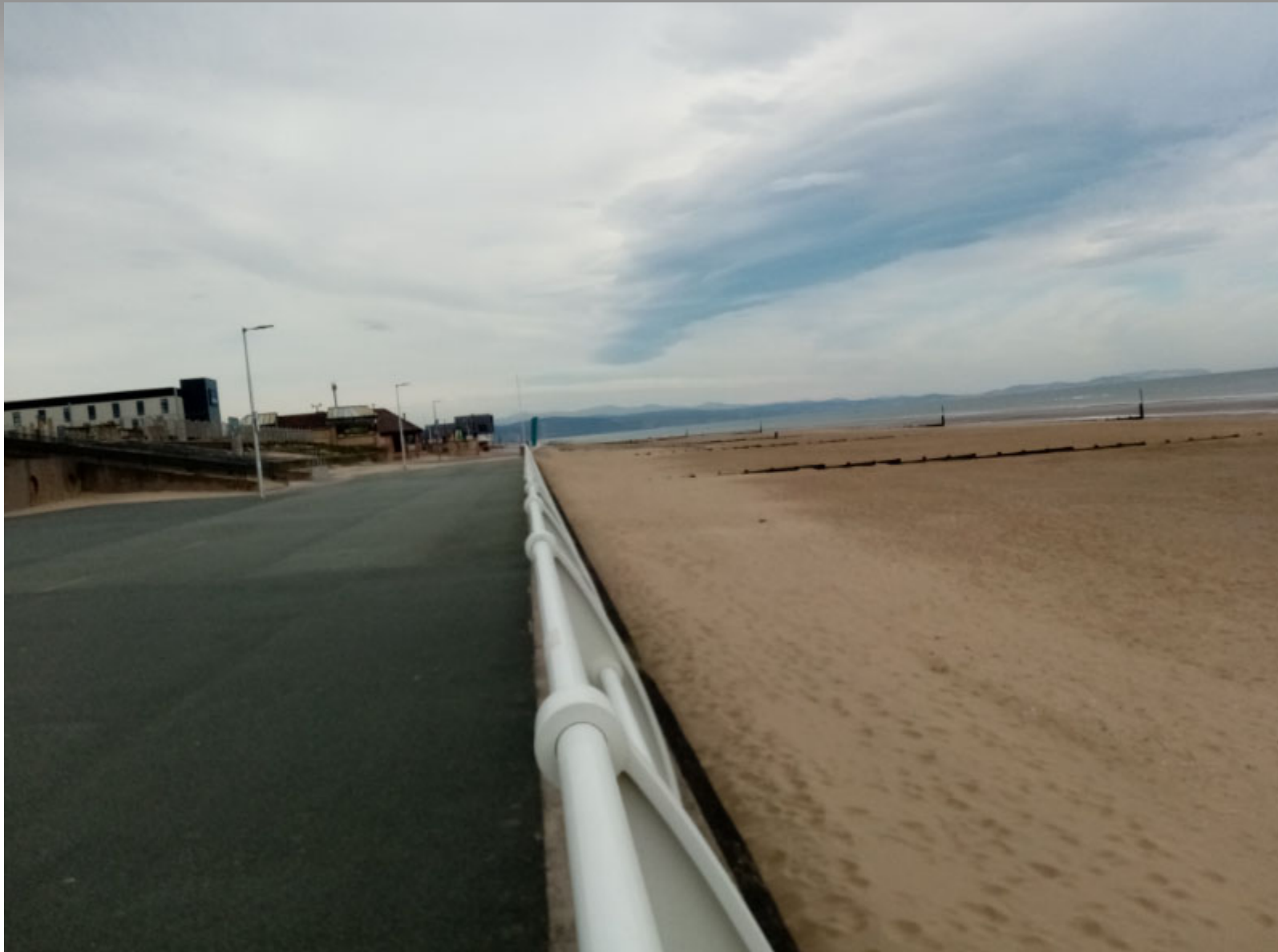
Existing promenade and defences
