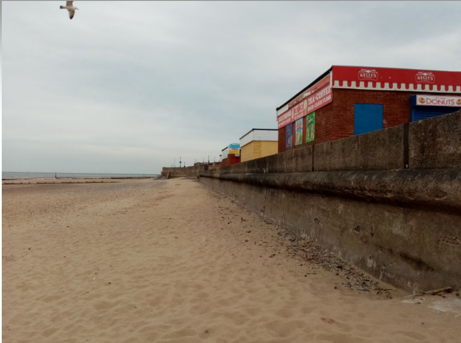
Existing promenade and defences
