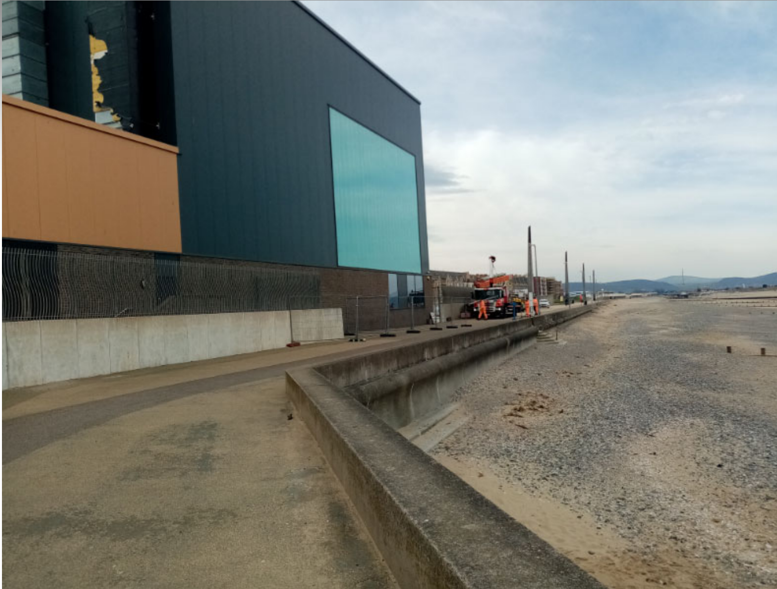
Existing promenade and defences
