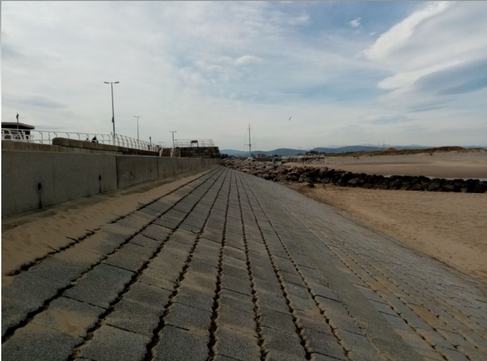
West Rhyl Coastal Defences (ramped & rock revetment)
