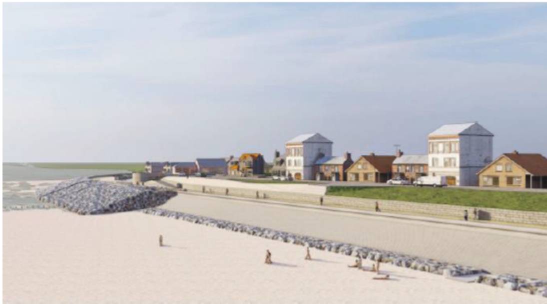
Figure 3-3 Visualisation for proposed rock scour protection (with possible future beach level)
