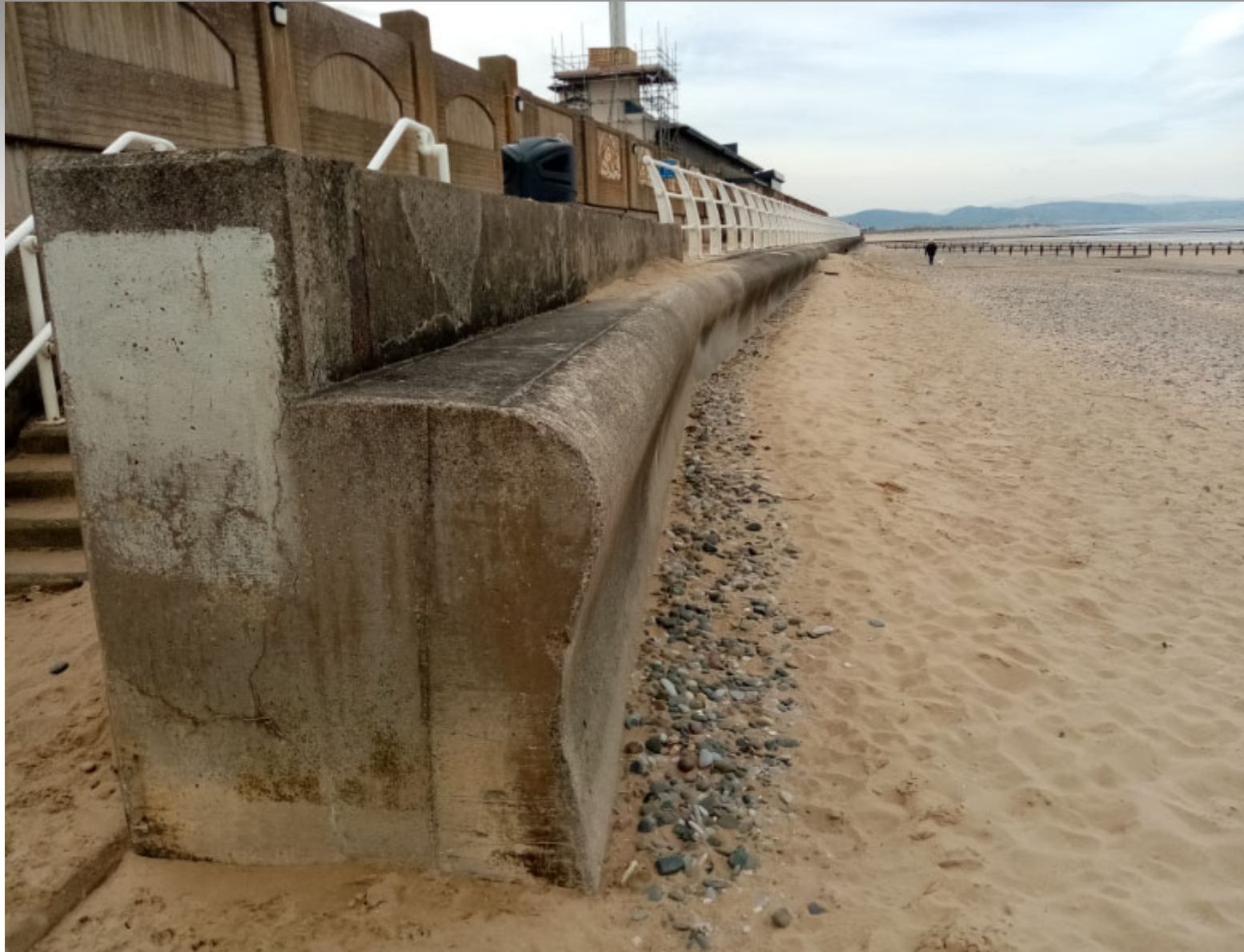
Existing promenade and defences
