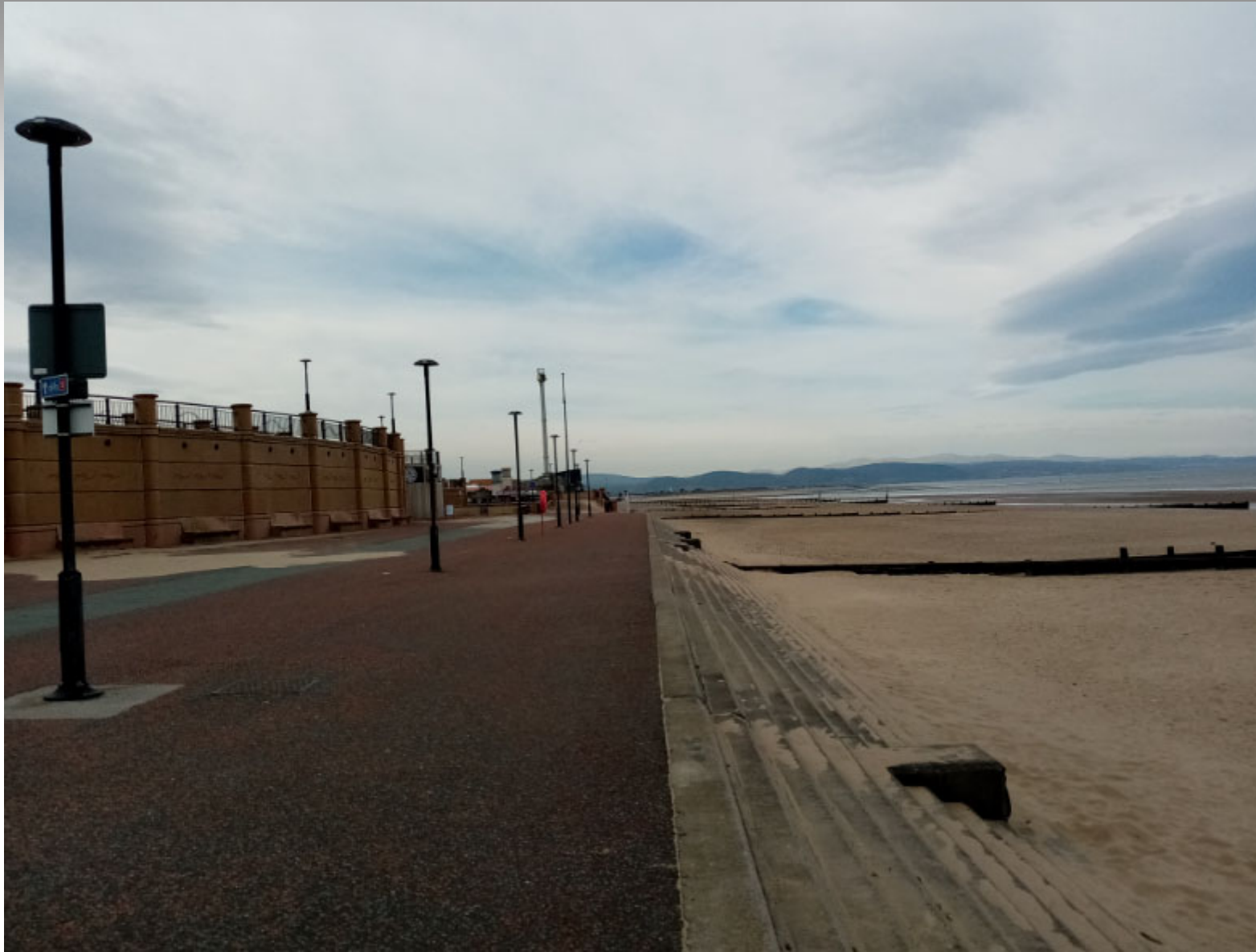
Existing promenade and defences
