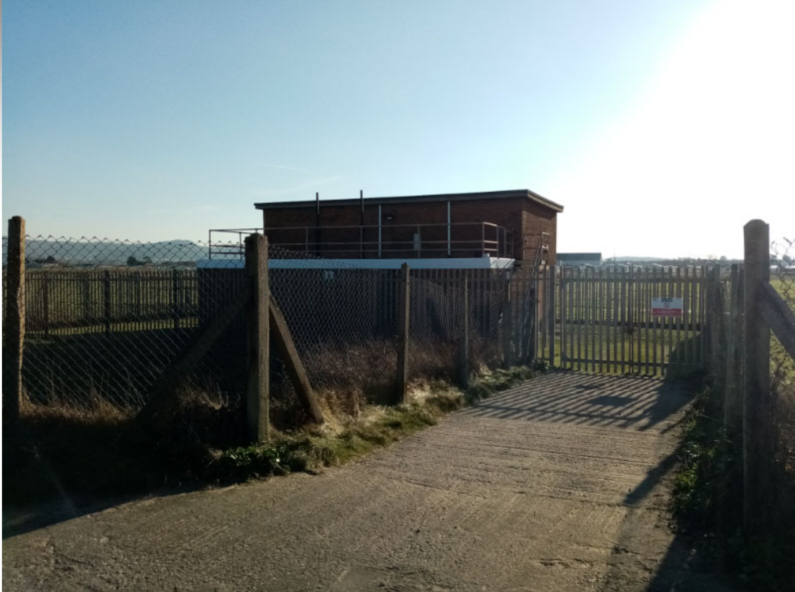
View of NRW pumping station from promenade
