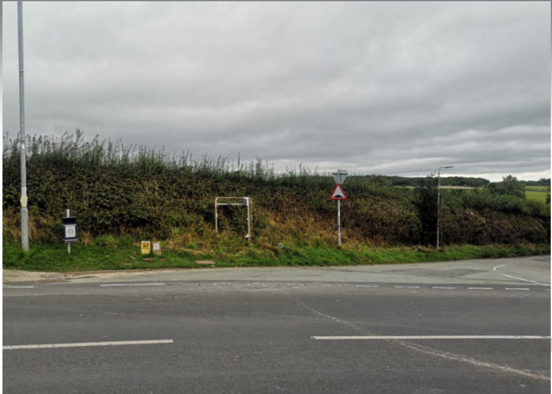
Site access from the top of Gwaenynog Road
