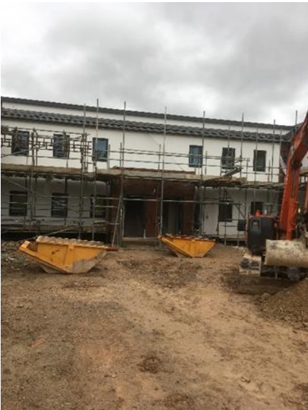
Figure 4: Awel Y Dyffryn, Denbigh Extra Care units under construction
