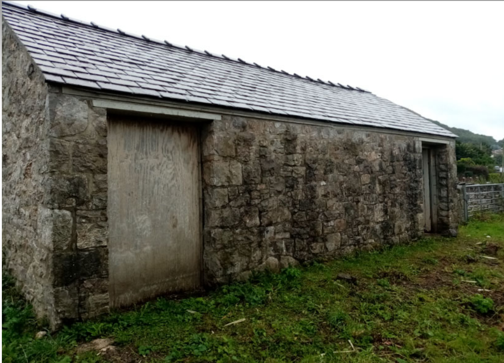
Existing agricultural building
