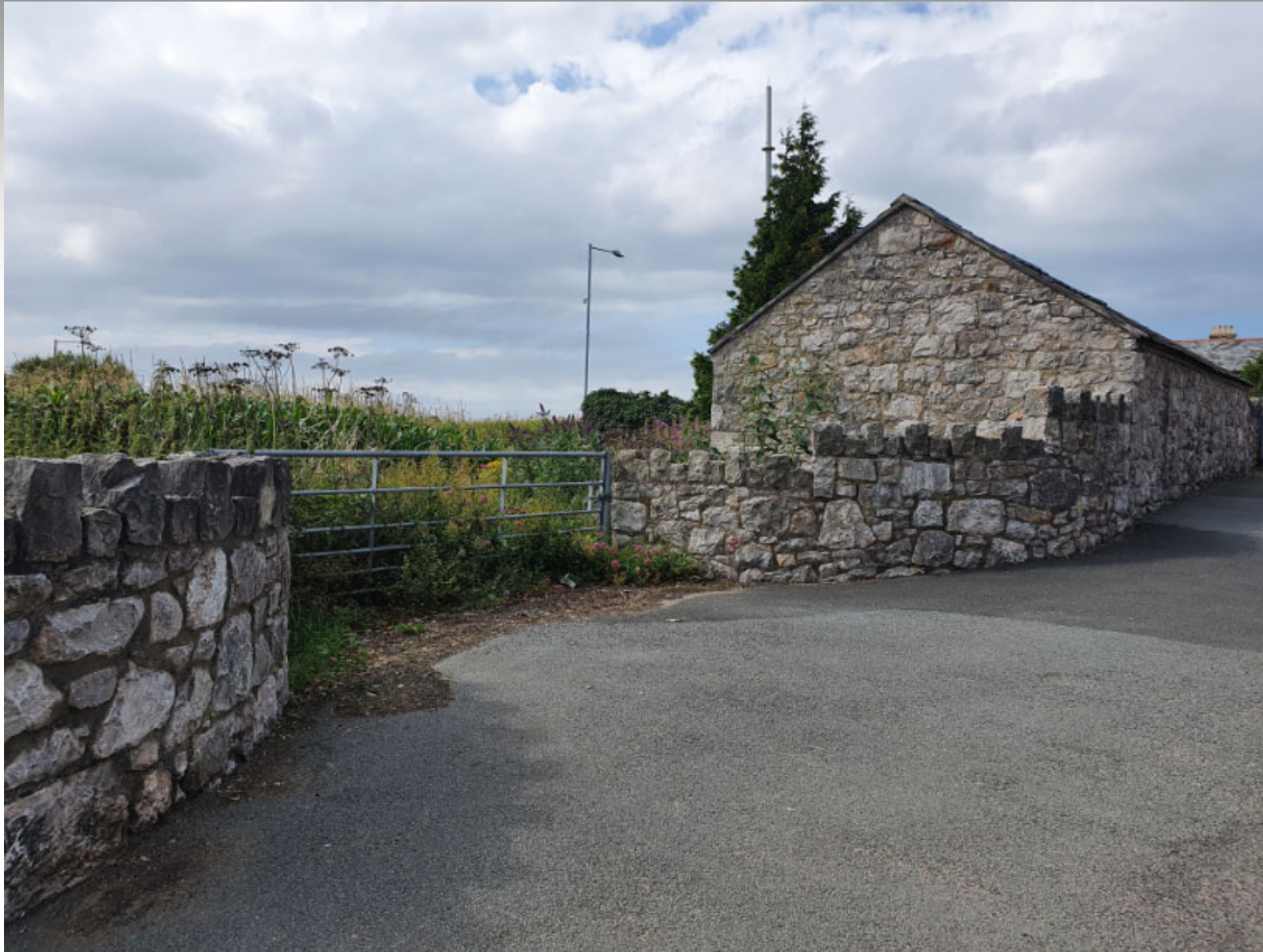
Existing agricultural building
