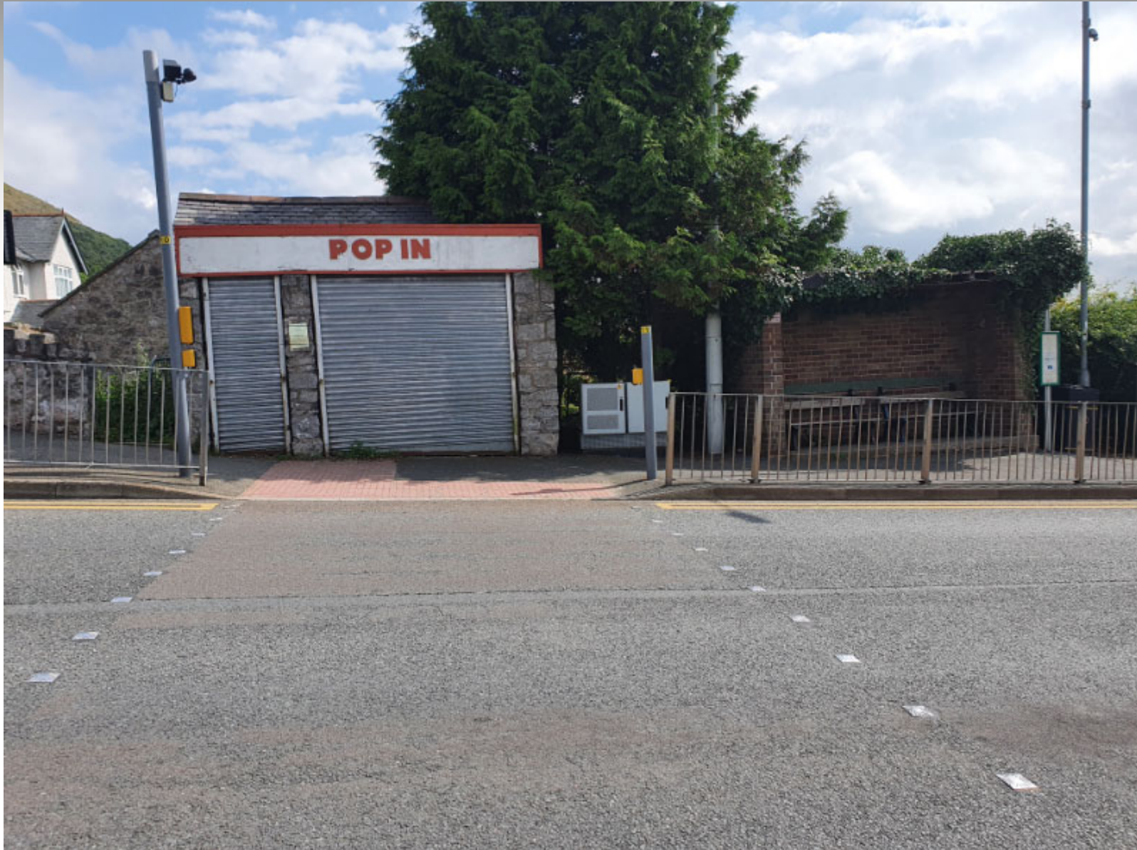
Existing 'Pop-in' retail unit
