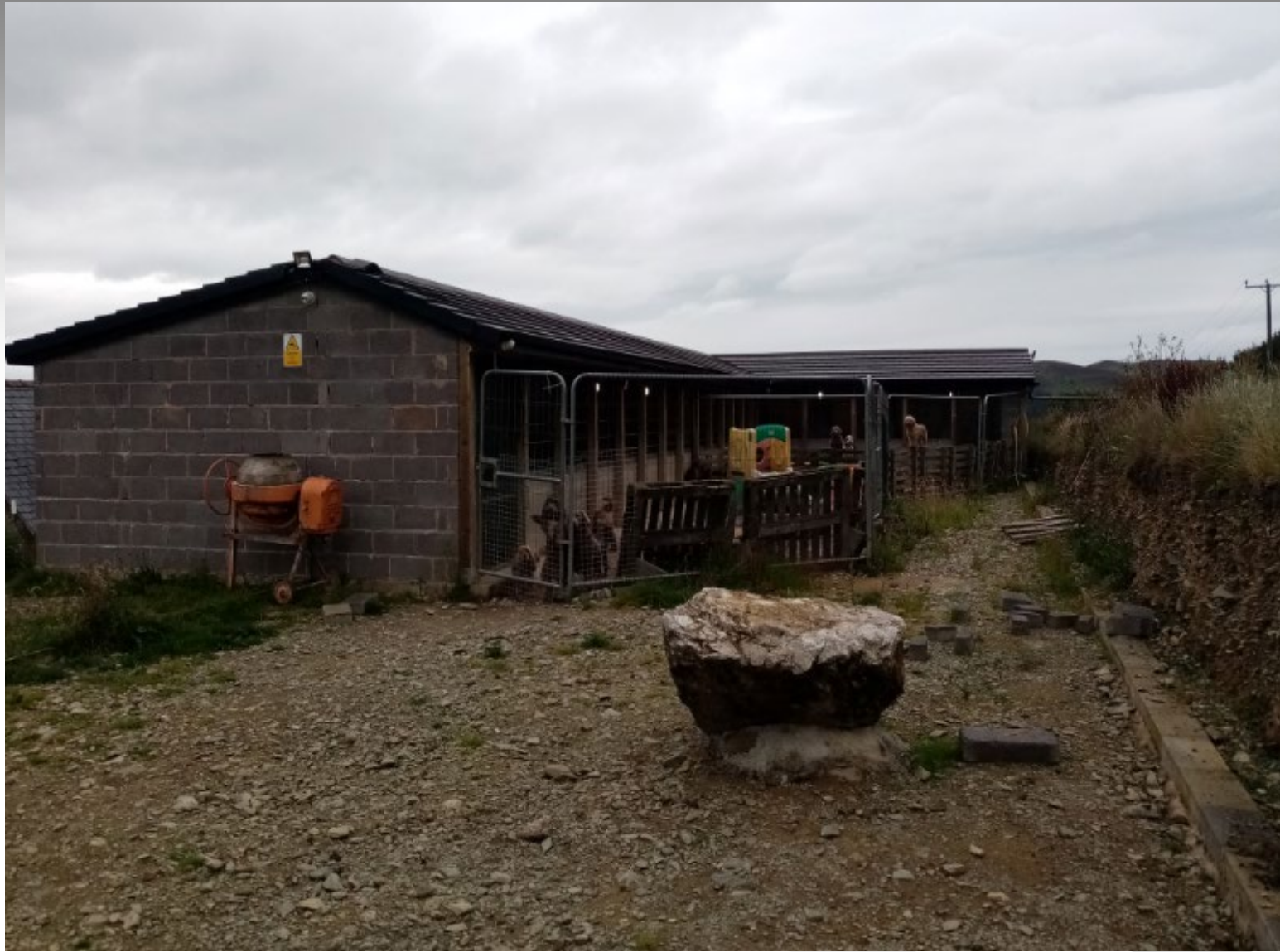
Photo of side and front elevation of kennels building
