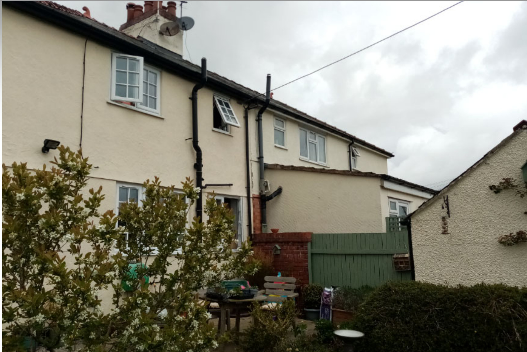
Rear of property and adjoining property
