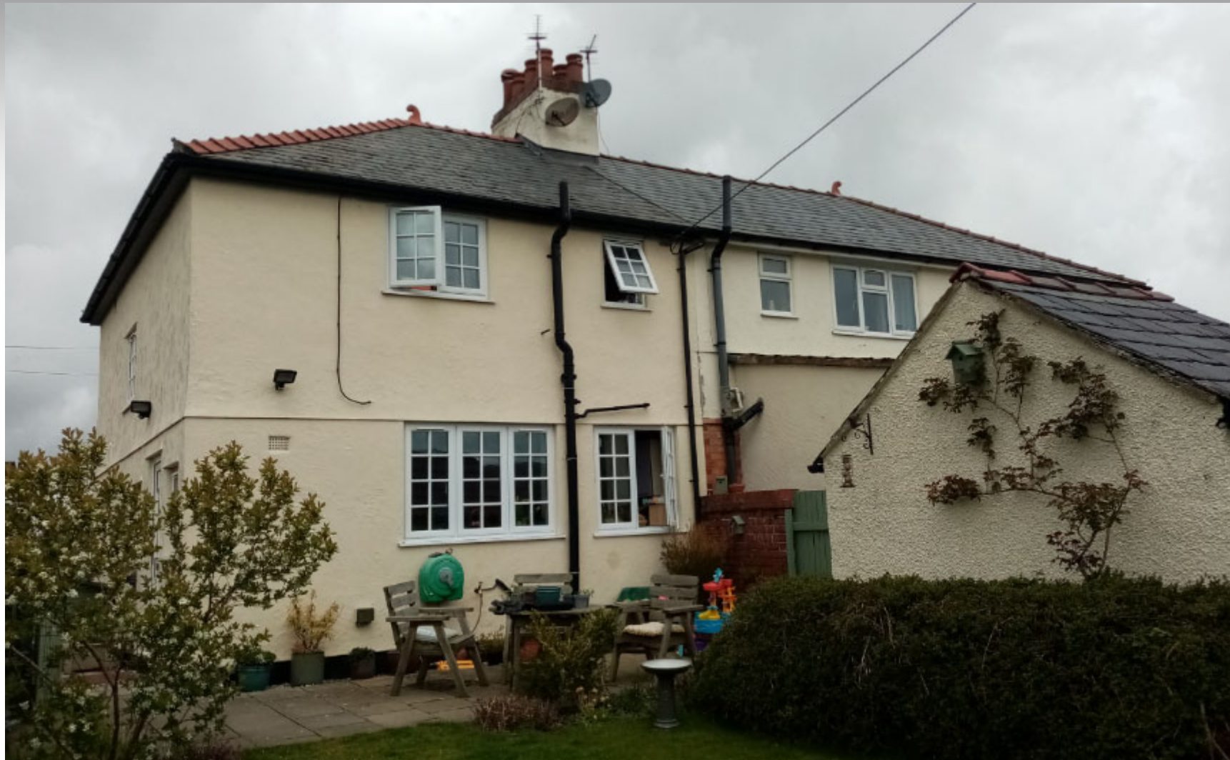
Rear of property and adjoining property
