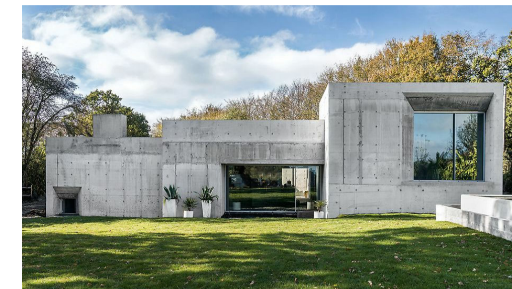
Concrete, lower floor
