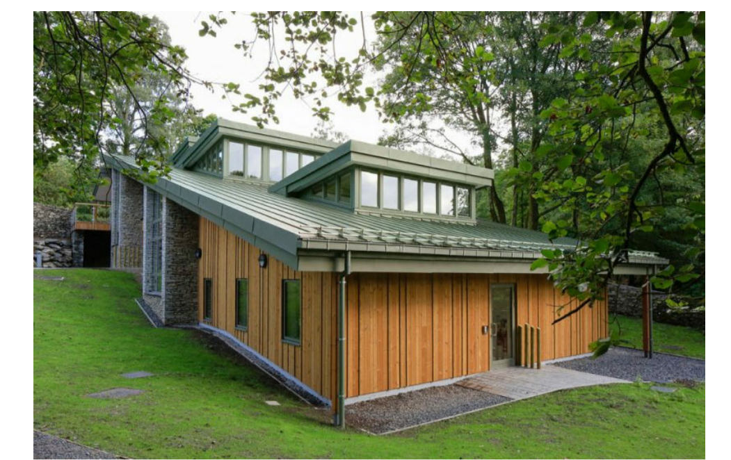
Zinc and Cladding
